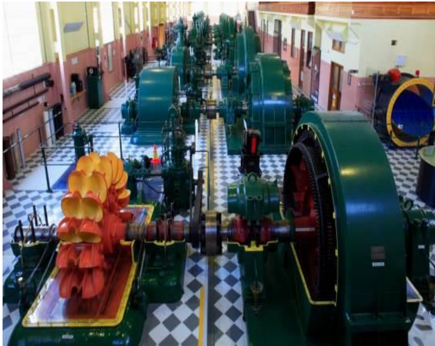
Figure 1. Turbines at the Waddamana Power Station in Tasmania. This power station is no longer in operation. It has been converted to a museum. Waddamana is a Tasmanian Aboriginal word meaning 'noisy water'.
